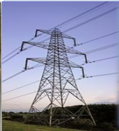
OPGW & UNDER GROUND Fiber Optic Link
